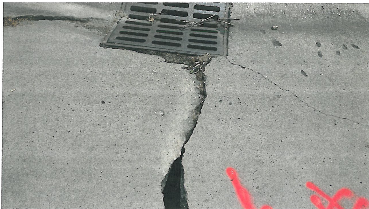
Corner catch basin is undermined
